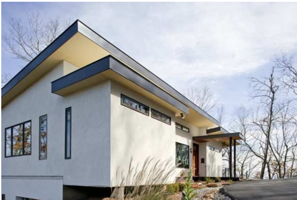
One of three houses in North Carolina built with Hempcrete, design by Push Design with Hemp Technologies; Photo: Push Design
